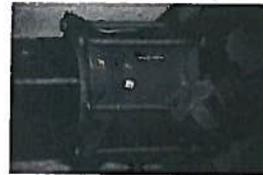
12. Stab coupling entirely onto IPS pipe.
