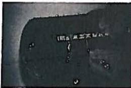
4. Mark each pipe 5" back from end. An additional 12" markback from each end will aid in inspection of the finished joint.
