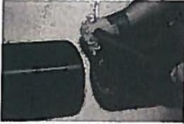
1. Clean cast-iron pipe end at least 6" back, removing dirt, scale, and oil.
