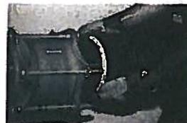
13. Hold spacer ring between pipes and slide coupling back over Cast-Iron pipe.
