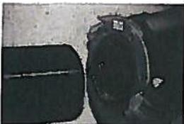
6. Slide locking plate onto CAST-IRON pipe with letter "A" facing IPS pipe.
