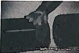
2. Clean plastic pipe end at least 6" back, removing dirt and oil. Pipe ends must be cut square and be free of longitudinal grooves.
