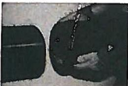
7. Slide Stainless Jaw Band onto CAST-IRON pipe with YELLOW MARK FACING LOCKING PLATE.
