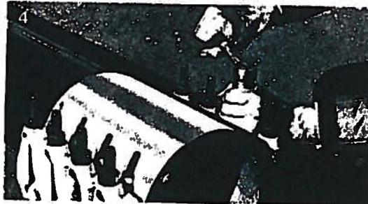
1. Clean pipe at break and wrap clamp around pipe. Clamp is easily opened by lifting bolts from slotted lugs. Installing Multi-Panel clamp is greatly simplified by unique design with captive bolt lug which keeps clamp in one piece during assembly.
