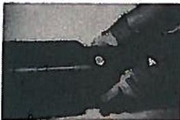
3. Insert properly sized metallic stiffener at least 7" long into plastic pipe end.
